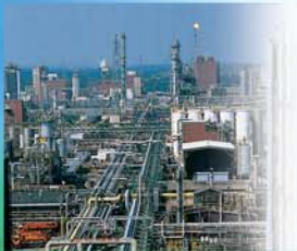
Chemical industry with pH measuring systems.
